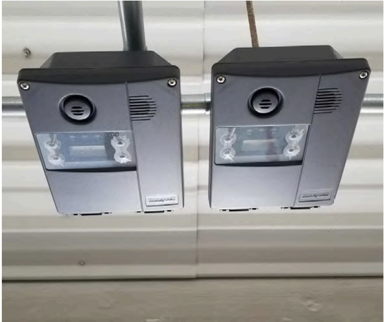
Upgrade Example: Methane Detection System Sensors
