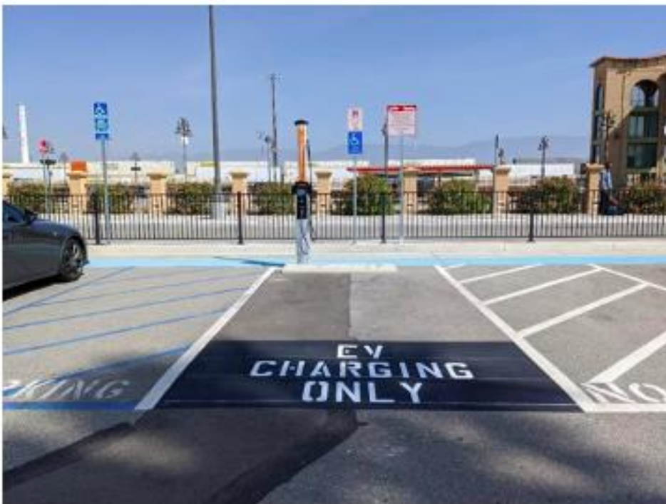
San Bernardino Metrolink Station ADA accessible single level two charger– Photo by Ivan Ramirez, SBCOG Management Analyst II
