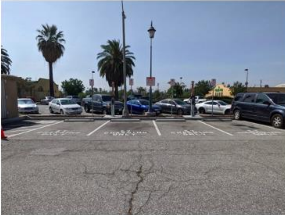
San Bernardino Metrolink Station dual level two chargers– Photo by Ivan Ramirez, SBCOG Management Analyst II
