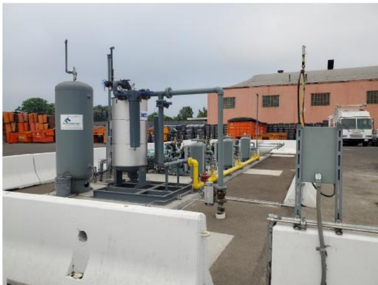
Picture 1. Station, looking southwest
